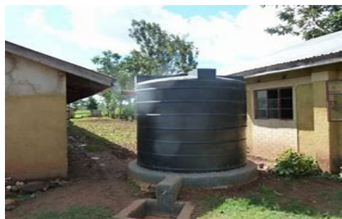
Components of Roof Catchment, and a roof water harvesting structure whereby rain is collected from two sides of the roof and directed through gutters to the plastic raised tank
