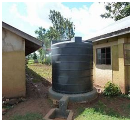
Figure 3.2: Components of Roof Catchment, and a roof water harvesting structure whereby rain is collected from two sides of the roof and directed through gutters to the plastic raised tank
